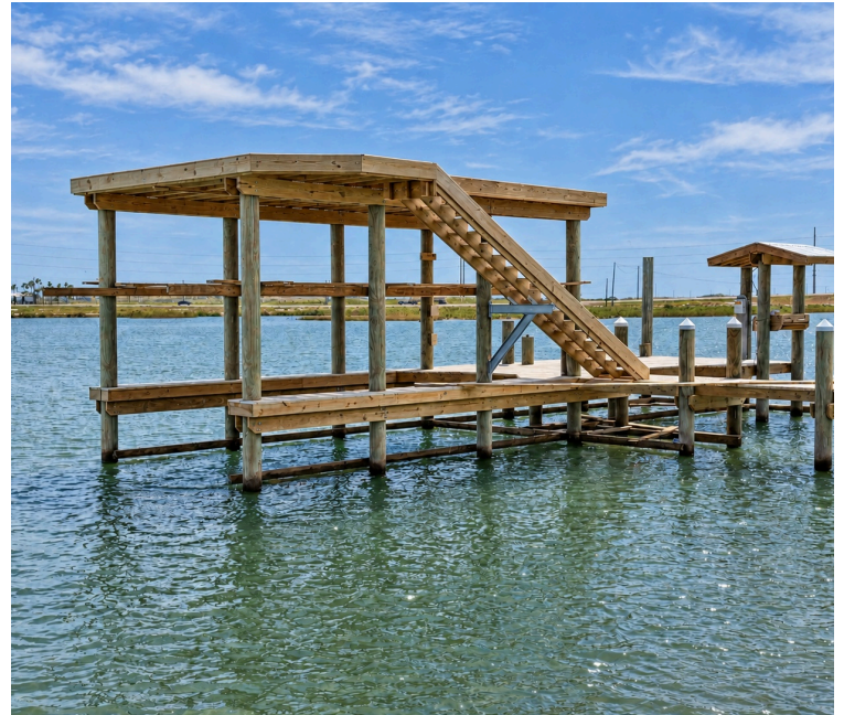
boathouse under construction
