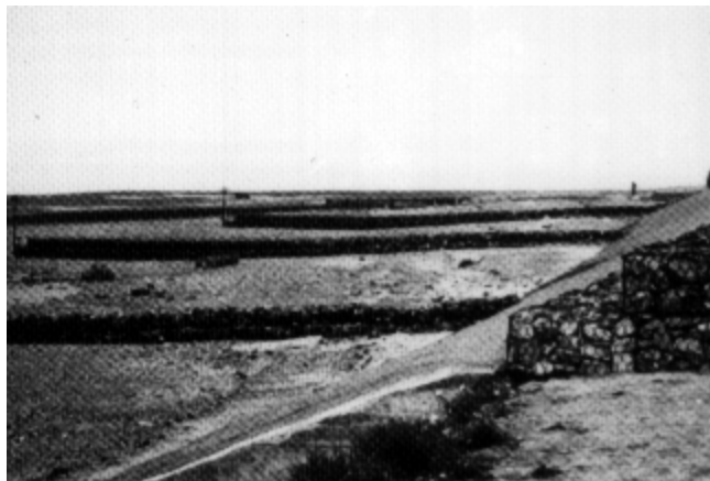
Figure 2-7. Gabion structure (revetments and groins)
