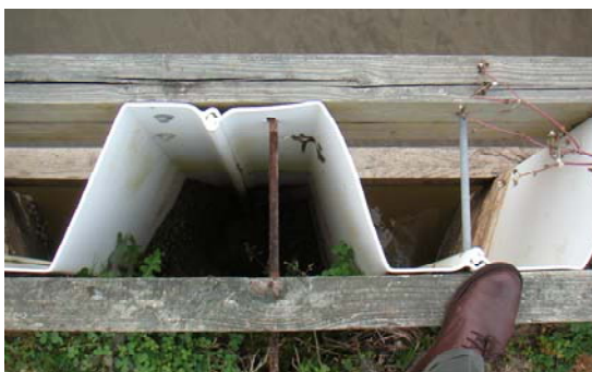
Figure 54b. Eight-year-old installations in Houma, Louisiana, Right bottom shows the eight-year-old unused sheet piles impacted with staple gun to show no cracking.
