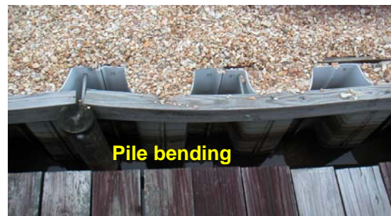
Figure 57. A relatively newly installed PZ 22 steel sheet pile showing onset of rusting
