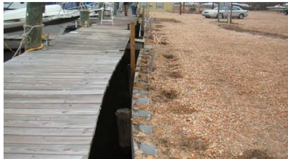
Figure 57. A relatively newly installed PZ 22 steel sheet pile showing onset of rusting
