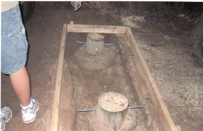
Finishing the foundations for each side with poles in ground for support
