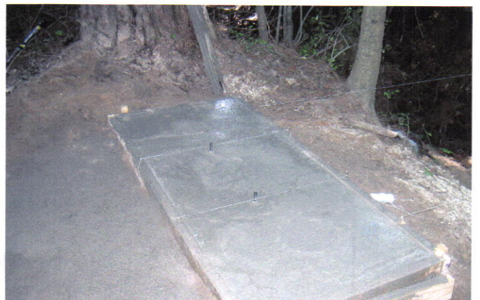
Finishing the foundations for each side with poles in ground for support
