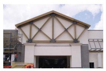
a truss that big in our facility, disassembling it completely [for shipment], and then reassembling it on the jobsite, without problems." After the trusses were built in the shop, they were pressure treated and then shipped to the jobsite in pieces, said Lincoln.
