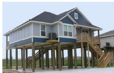
Gun Barrel pilings, about the same cost as square timbers, are stronger and have better storm surge properties.
