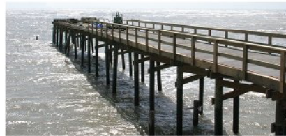
The pilings for this Texas coastal pier are treated for use in saltwater (treated 2.5 pcf with CCA).
