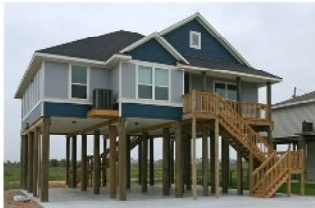
.60 CCA is often used to treat house pilings such as these no-taper Gun Barrel pilings installed by a Texas shoreline.
