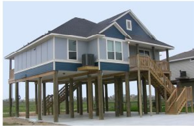
Gun Barrel pilings are stronger than square pilings and cost less but deliver the same uniform appearance.
