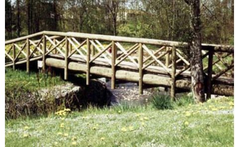
Bridge Timbers & Poles
