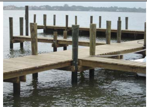
Treated Pilings & Decking
