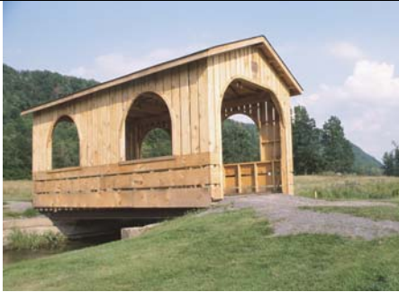
Bridge Timbers and Materials
